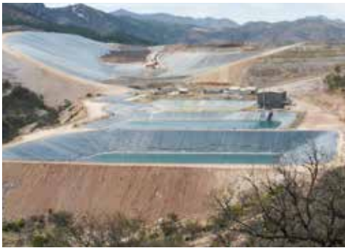
Heap leach facility at Alamos Gold's Mulatos Mine in the Sierra Madre Occidental mountain range, Sonora, Mexico.
