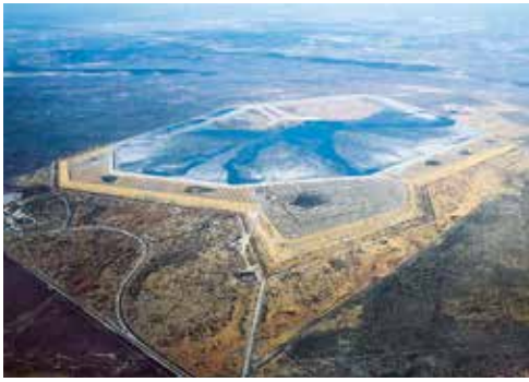
The staggering size of many modern tailings storage facilities qualifies them for that exclusive list of man-made structures visible from space. They share many similar characteristics with heap leach facilities – the modern versions of the gold cyanidation operations pioneered by De Beers in the late 1800s.
